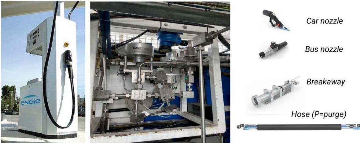
**Figure 2.2--1. Typical arrangement of a high pressure H2 dispenser**
