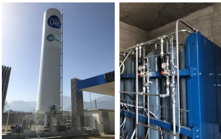
Figure 50 - LNG Vertical tank (left), CNG storage (right).
