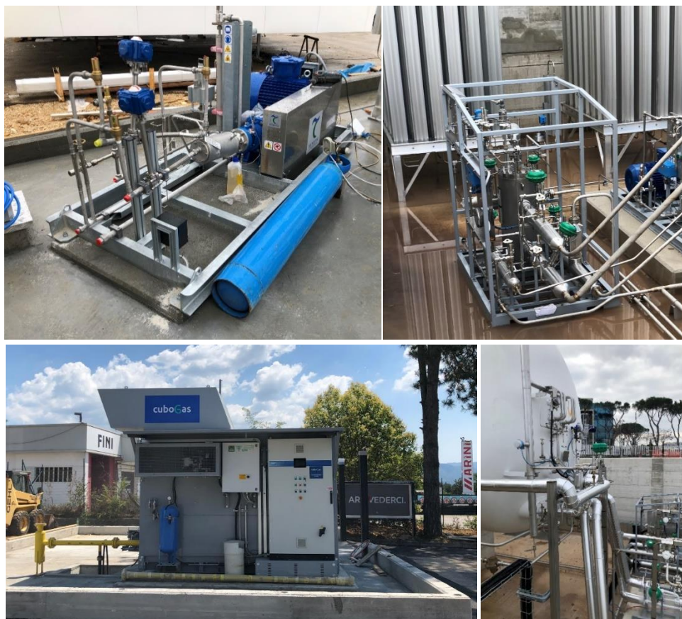
Figure 49 - Cryogenic high pressure pump (top left), cryogenic LNG pump (top right), CNG compressor (bottom left), L-CNG Tank connection (bottom right).
