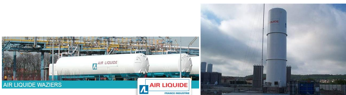
Figure 21 - Horizontal and vertical liquid hydrogen storages.
